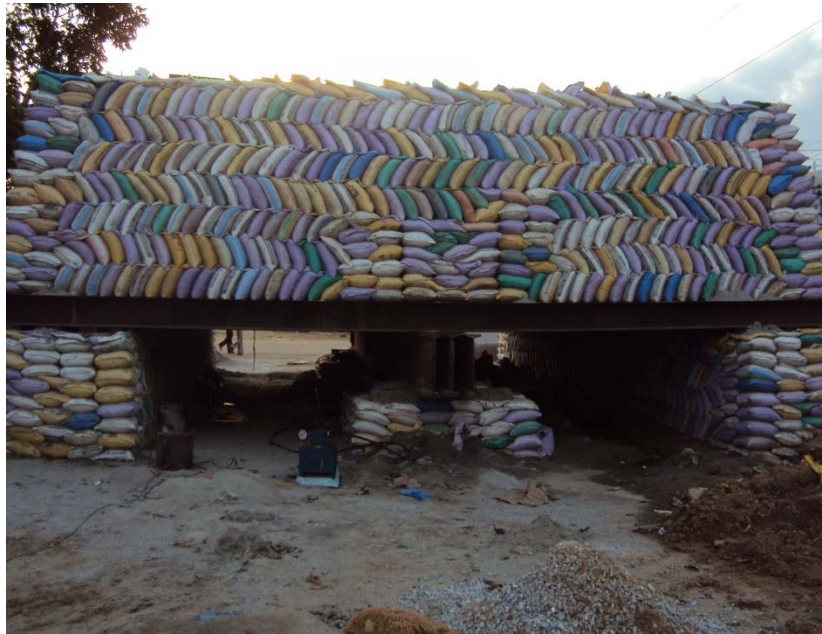
Fig. 7.4 (a): Pile load Test Setup
