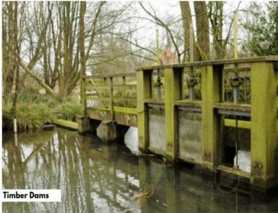
Fig. 11.12. (a) Framed timber dam (b) Beaver timber dam.
