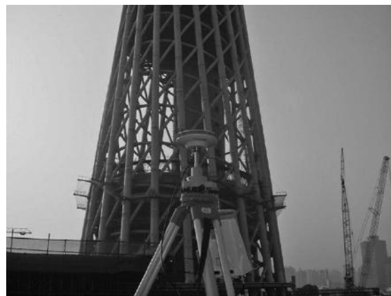
Figure 3: Global positioning system (GPS, Leica Geosystems Model 1230) used in construction monitoring of Canton Tower.
